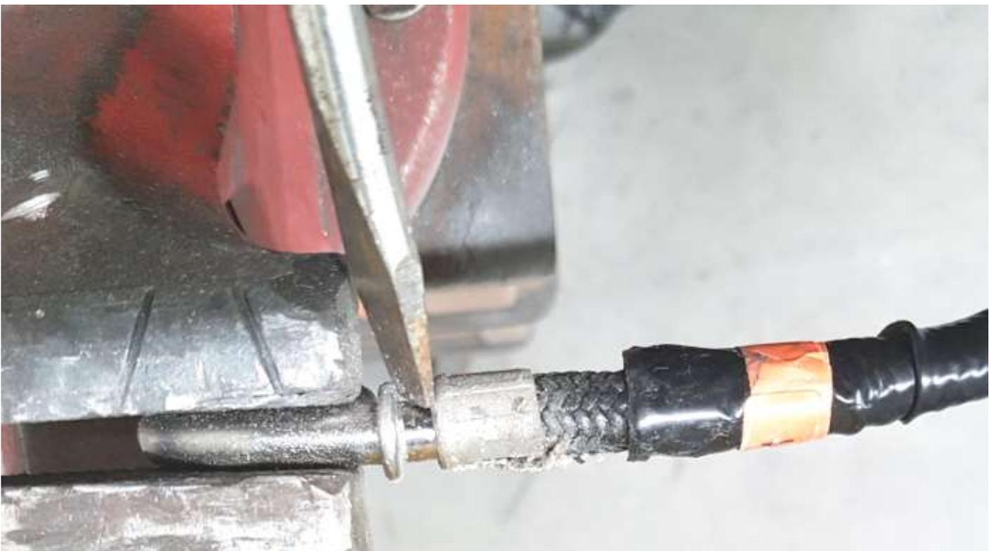
**Install the new fuel hose and fix it by the clamps.**
